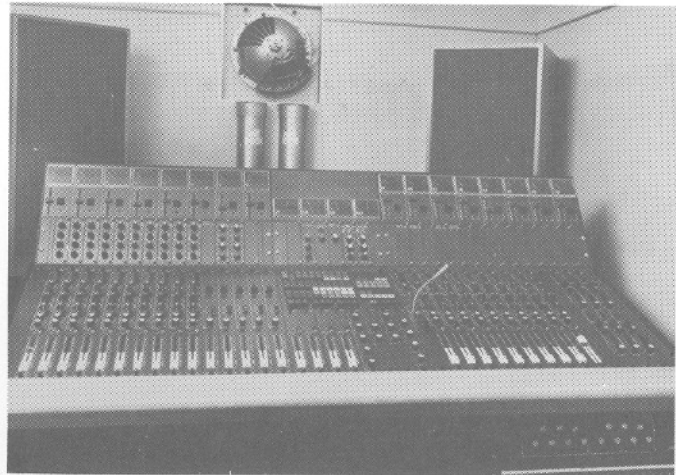
FIG. 8 Part of the inside of the IBA's mobile control room which was specially equipped for surround sound broadcasts. Courtesy IBA.
